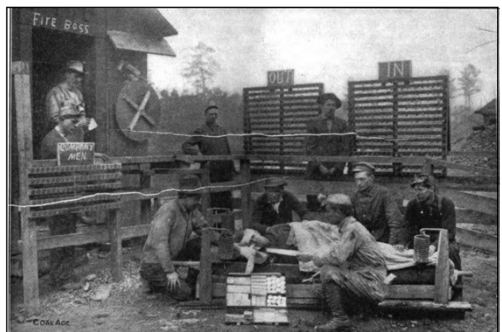
Wooden frame stretcher designed to be placed on a mine car to remove an injured man. Safety was a never ending effort for the company as mining is a dangerous occupation. Other features are checking with Fire Boss for gas. (Coal Age 1914, courtesy of Thomas Denney)
