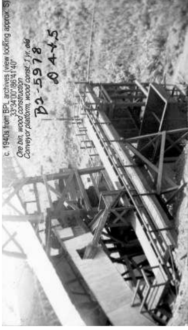
c. 1940s from BPL archives (view looking approx. W) 33-34100-864140 Conveyor housing, wood frame, corr. iron sides & roof, pine floor, average 10 ft. above ground on wood piers B2-5978 002
